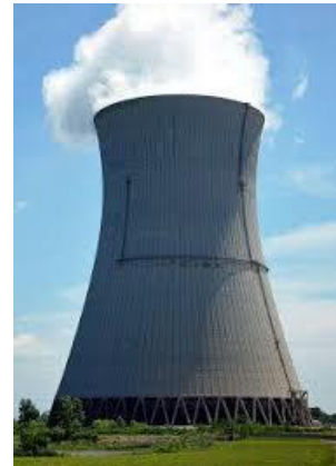
Fig 8.3 – Nuclear power station cooling towers
